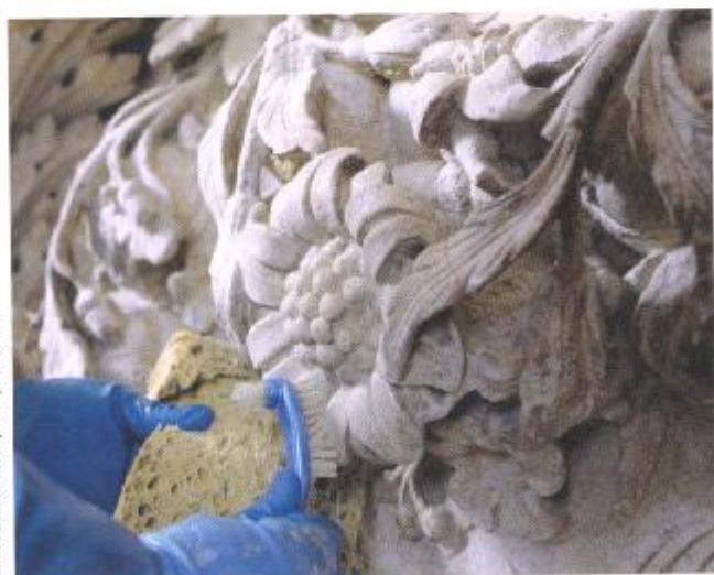
Washing of intricate carved detail after removal of Arte Mundit
