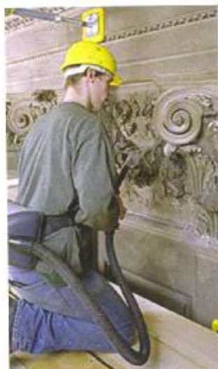
Removal of significant deposits of dust using vacuum
